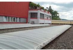
These continuous barrel T-Vault rooflights are designed to be both functional and affordable. With widths of up to four metres and unlimited lengths, our T-Vault rooflights are suitable for a range of flat roofs.
