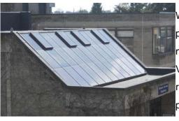
With a width of up to six metres and unlimited length, these purpose-made, flat roof skylights are designed to bring as much natural light into a building as possible. Our Em-Vault continuous rooflights – also known as barrel vault rooflights because of their shape – can be used on single ply, felt, hot melt, asphalt, liquid, GRP and lead roofs and can be made to virtually any specification.
